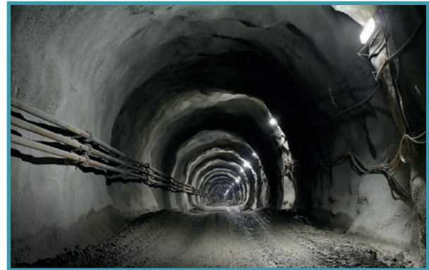
Shotcrete Application in Mines
