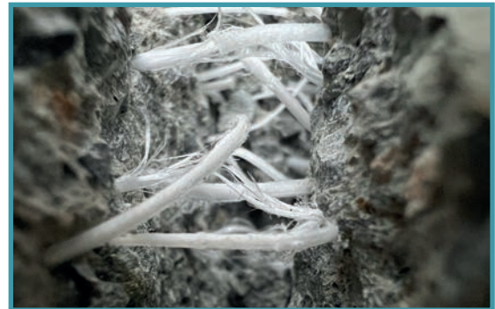
Appearance After Plaque Fracture Test
